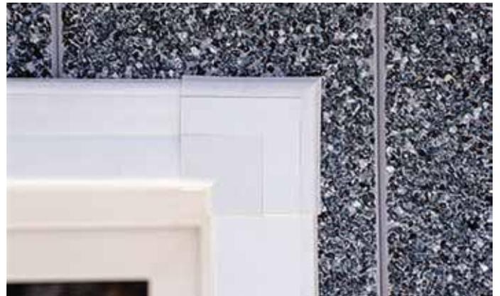
*The click and ready principle of vinyCom saves time-consuming cuts and fixings. Thanks to the vinyCom system corners, the reveal corners fit accurately to the millimetre even without mitre cuts. The cover strips are available in different colours. This lets you put colourful highlights on windows and doors.*
