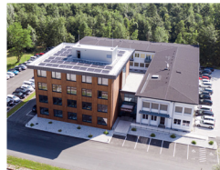
binderholz TimberBrain Office Building, Hallein | Austria
